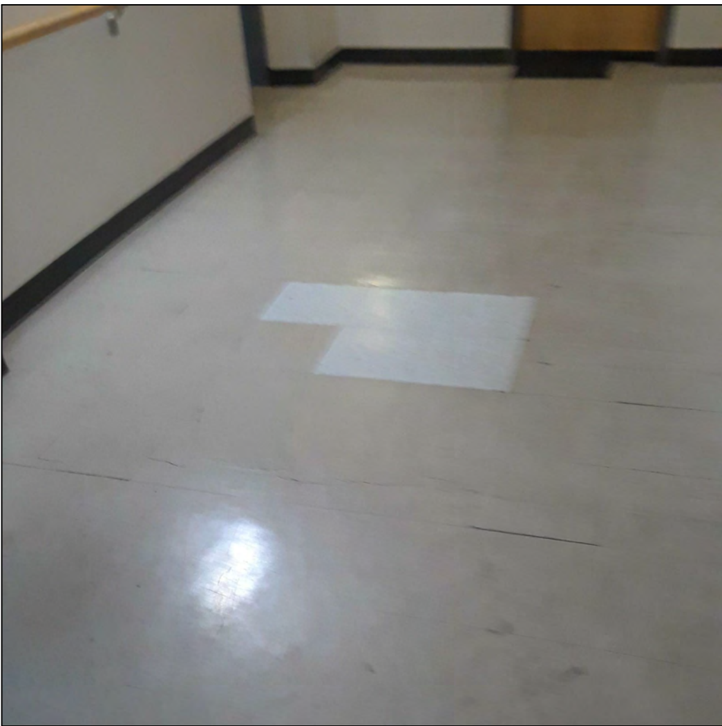
02 - Main hallway view
