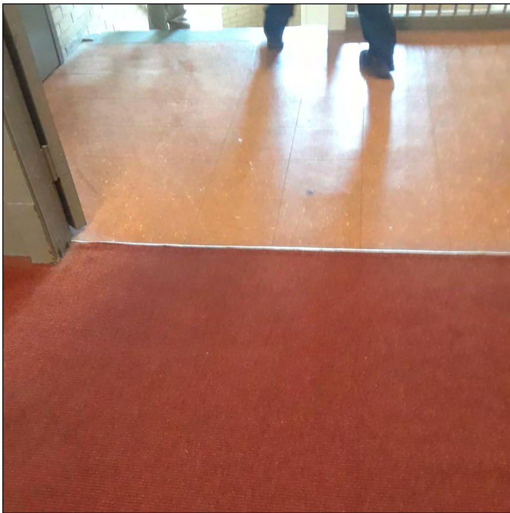
05 - Main hallway to landing
